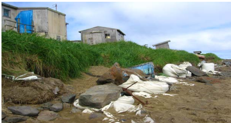
Photo 3: Sandbags for erosion protection front a small portion of Mekoryuk, August 2007.
